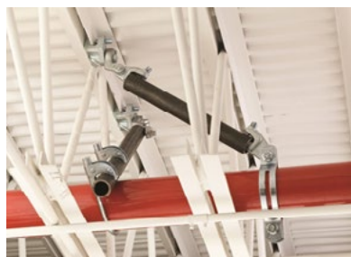
PINCE DE POUTRE TYPE SOLIVE SUPPORT
