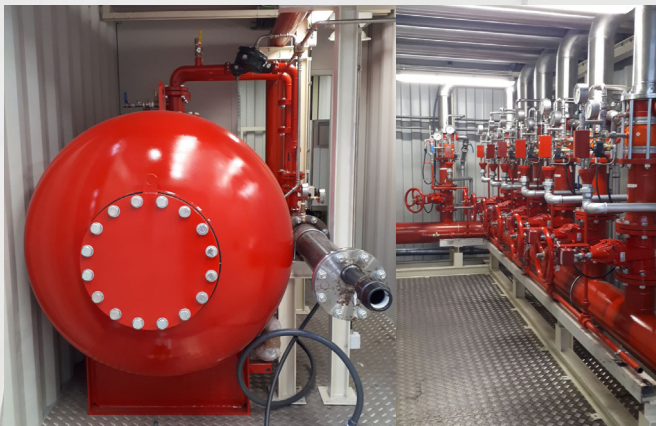
Deluge valves with trim. Foam storage and mix control room
