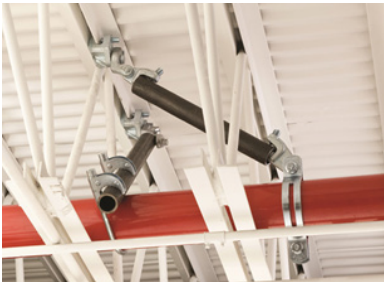
BAR JOIST ATTACHMENT
