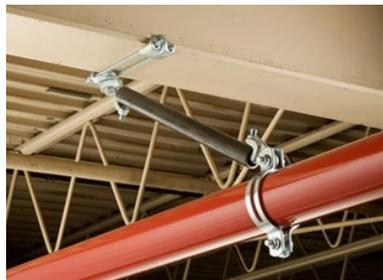
**FIJADOR A VIGA TIPO I AJUSTABLE**
