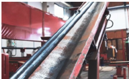
Pipe cleaning and dimensional control.
