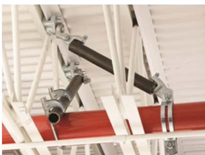
Bar joist attachment.
